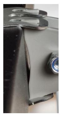
Remove the four Allen screws from the square metal plate. Press the two side plates (hook anchors) against the frame so that there is space between the frame and the clamp on the other side. Slide the square metal plate in between until it is nicely centred in the clamp.
